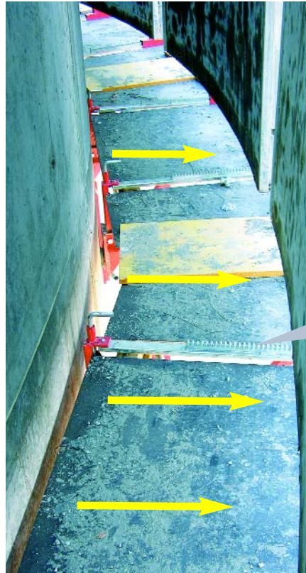
View of the track for the rack and of the shim that secures the overall unit during form removal.
